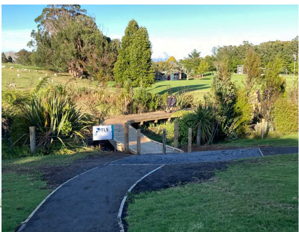
Example of stream enhancement and protection at Tangaroa
